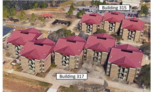
Figure 2. Buildings 315 and 317, Ft. Gordon, GA
